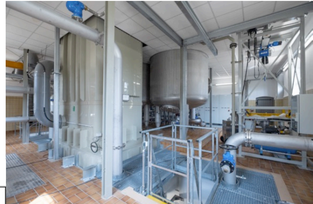
Energy intensive reverse osmosis facility to eliminate PFAS at the Rastatt test site to make drinking water potable
